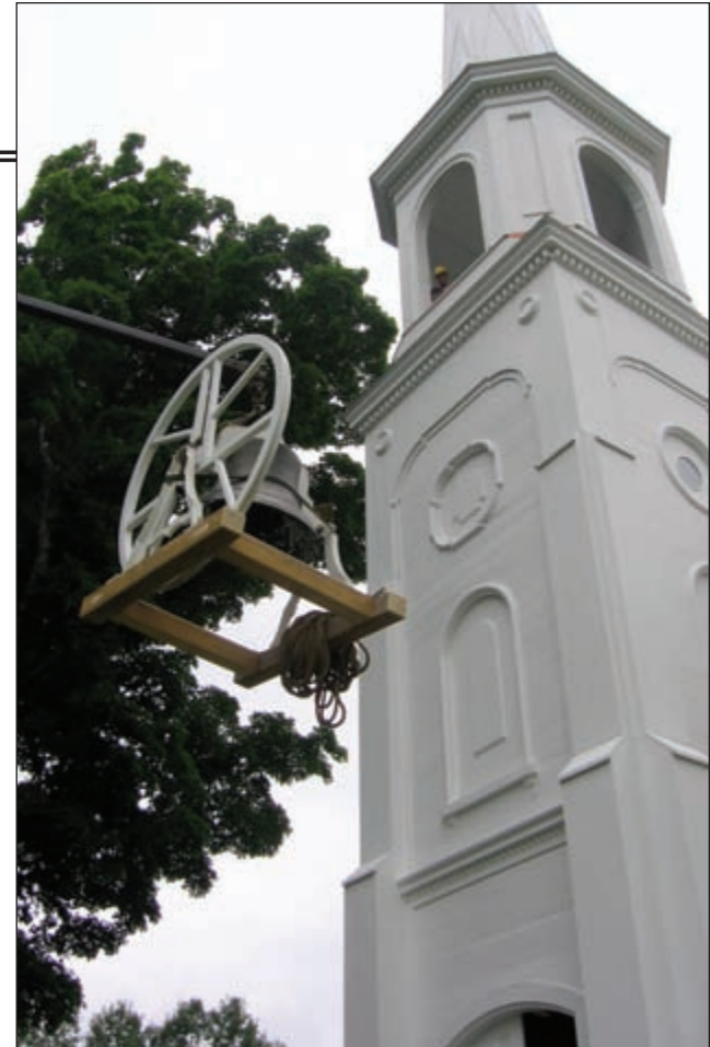
The bell of the North New Portland Community Church is lifted back into the belfry after both it and the church had major renovations and repairs done.
